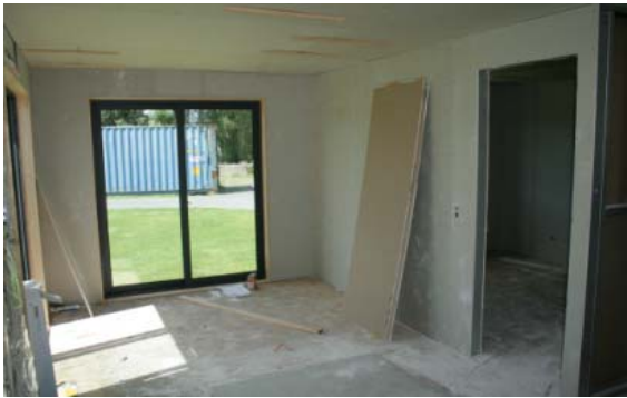
Interior plasterboard installation
