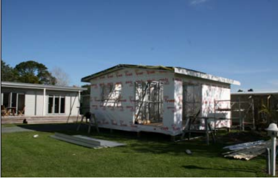
Colorbond Roofing done
